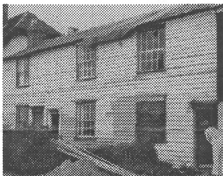
The cottages in the process of being converted into our Clubhouse
